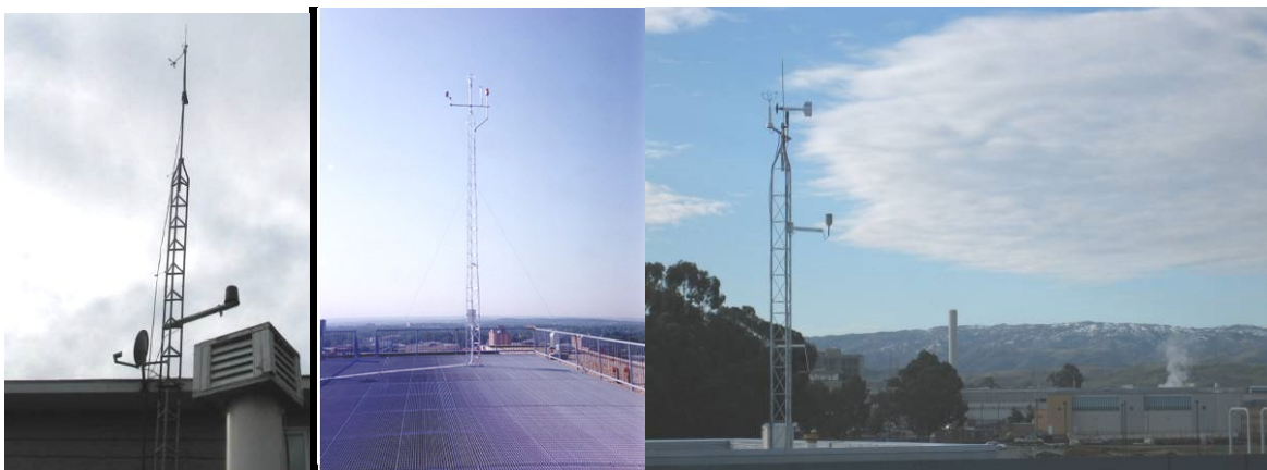
Figure 4. Example rooftop towers
