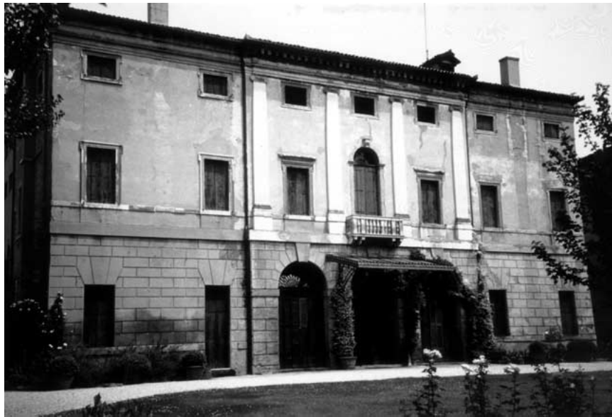
Figure 2a. View of the SW facade of the Poleni House facing the garden. On the right, the Bovetta Channel has now disappeared, covered with earth. On the ground floor, in the middle, the three arches of the loggia, i.e., the Summer Room. On the left, the Physics Laboratory. On the first floor, on the right, the last two windows are of the Library where the Amontons thermometer was located.
