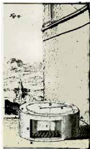
Fig. 5 Twisted cord hygrometer with rotating pointer built improving the idea by Sanctorius. (D'Alancé, 1707)
